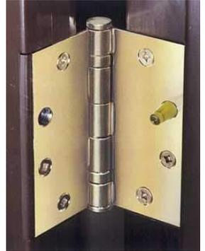
Once this is complete, as the door closes, the pin in the jamb will penetrate the hole in the door and the door will be held in position even if the hinge pins are removed.
